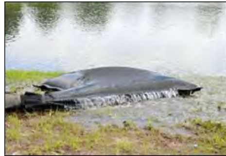
Plate 4-6 Silt bag under inspection
