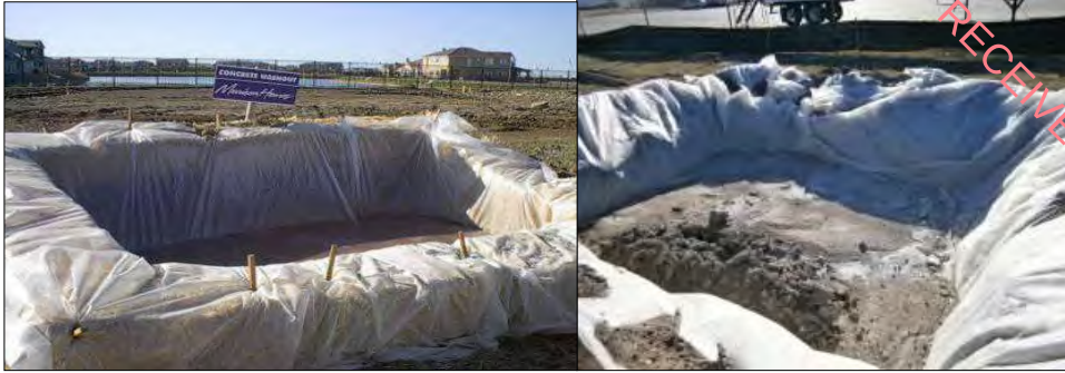
Plate 4-3 Concrete washout area
