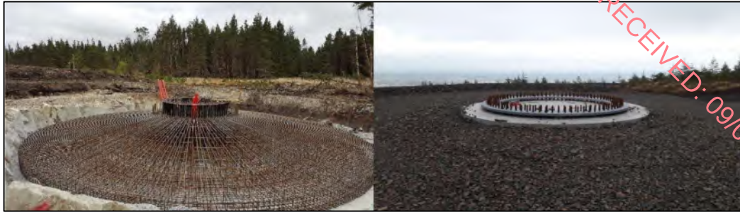
Plate 4-2 Turbine Foundation Anchor Cage surrounded by reinforcing steel and finished turbine base
