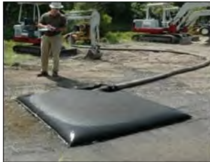
Plate 4-5 Silt Bag with water being pumped through
